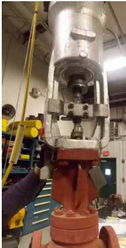
Hydraulic actuator attached to a process valve.
