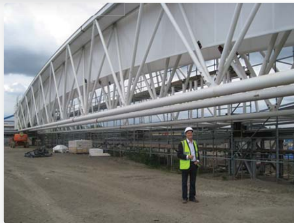
John Westmucket, structural engineer and then director of engineering design firm Edge Structures Ltd., London, England, stands under one of the test roof trusses. These trusses were later installed at Wimbledon.
