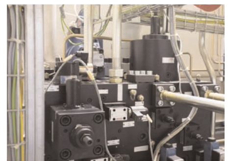
Installation in the Press
