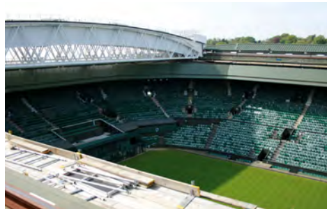
Wimbledon Centre Court view at roof level.
