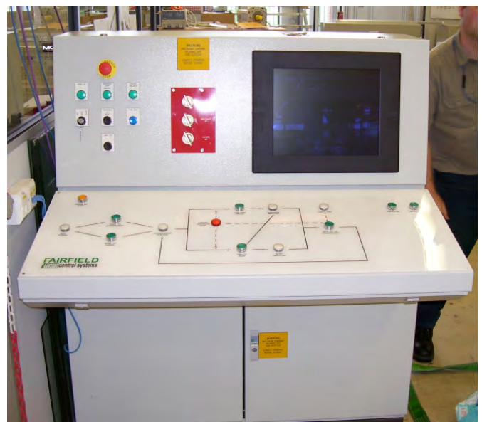
Main Control Panel in test
