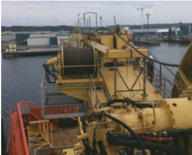
Crane Hoist Winch
