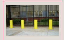
Bollards This type of barrier is more aesthetically appealing than the large plates and also allow pedestrian traffic.
