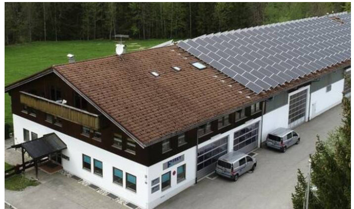
Frey and Co. facilities, Lenggrries Fleck, Southern Bavaria, Germany (photo courtesy of Frey and Co.)
